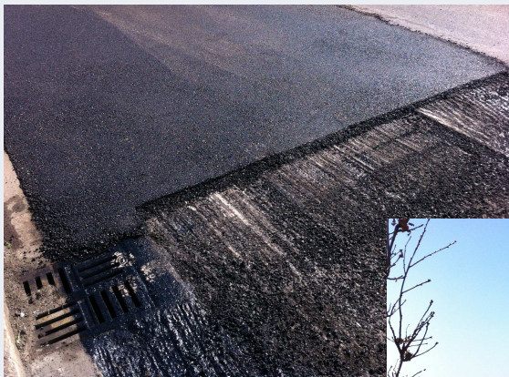
Noise absorption asphalt at Prato
