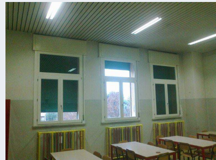
Noise barrier installed at the primary school "Lattes" at Vicenza
